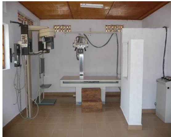
Finished x-ray room
