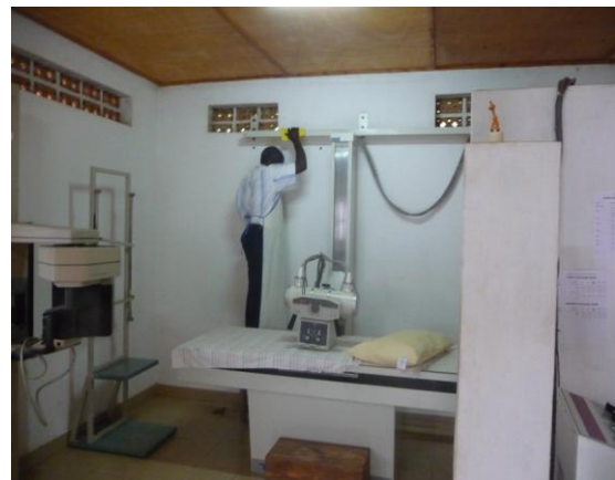
Ezra cleaning the electrical equipment
