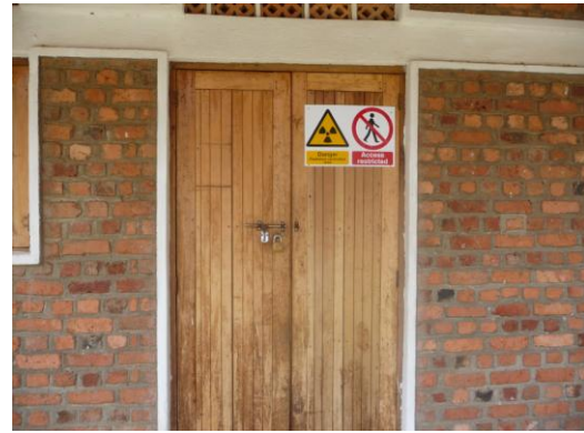
New radiation warning signs
